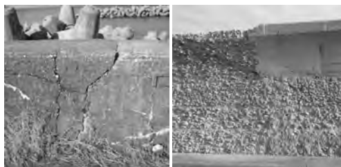
Fig. 1 State of deterioration of concrete at fishing port.
