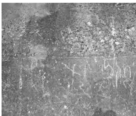
Fig. 15 State of concrete surface at Odawara fishing port.
